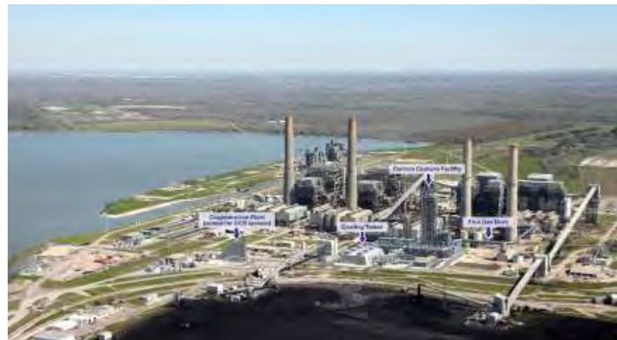
NRG Parish, USA
