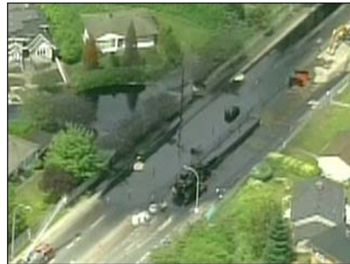
15 th January 2009 Vancouver- line rupture
