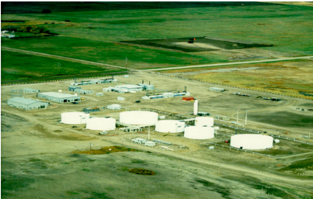
Figure 8 Weyburn oil field control centre (Courtesy of PanCanadian)
