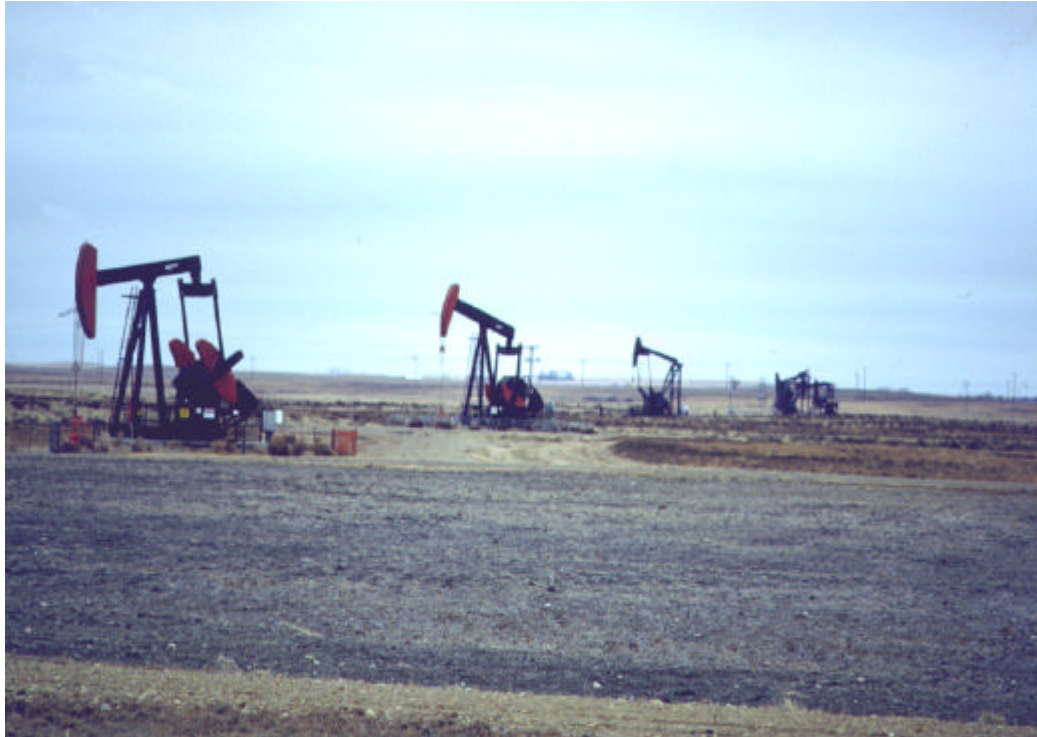
Figure 6 Production Wells on the Weyburn Oil Field. (Courtesy of PanCanadian)
