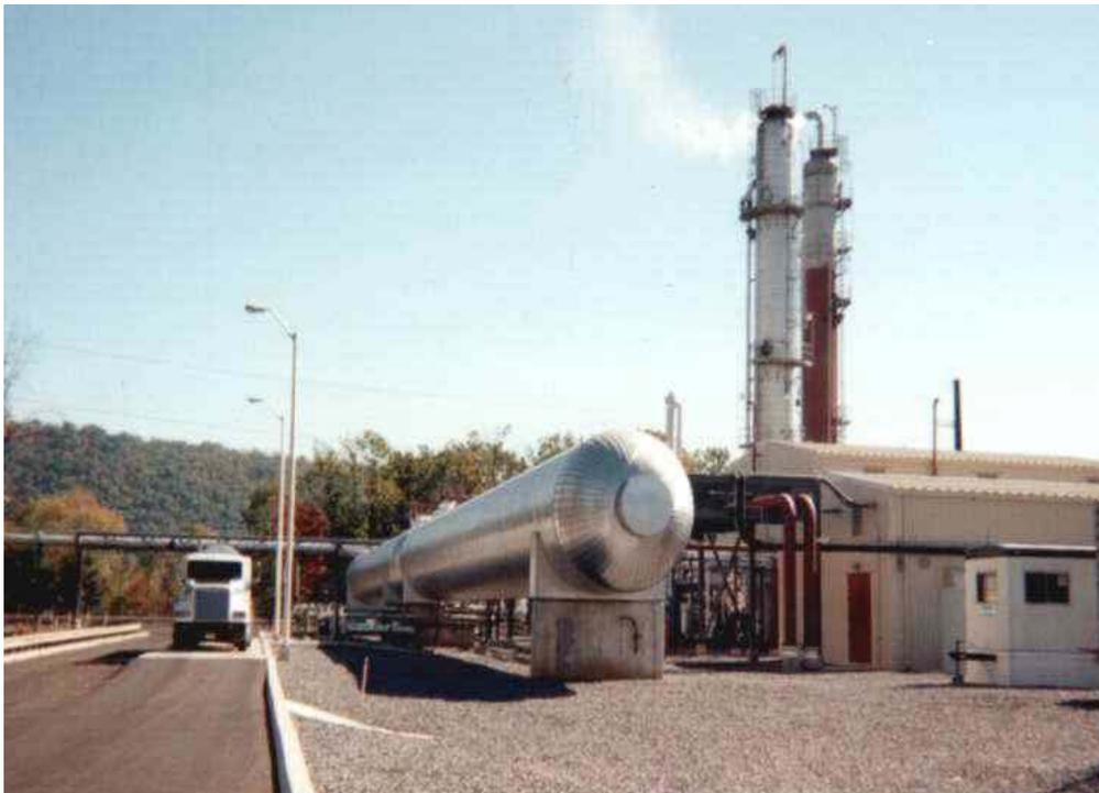
The photograph illustrates the CO<sub>2</sub> capture facility. Two horizontal CO<sub>2</sub> storage tanks can be seen. The 2 vertical columns are the CO<sub>2</sub> absorption column and the CO<sub>2</sub> recovery (solvent regeneration) column. The CO<sub>2</sub> system includes a solvent reclaimer. The majority of the plant is built in carbon steel with stainless steel used in
