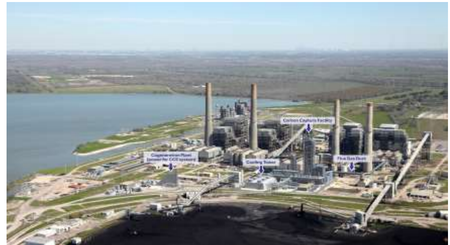
NRG Parish, USA
