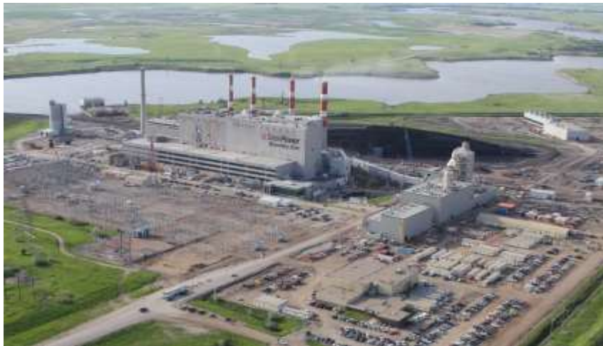
Boundary Dam 3, Canada
