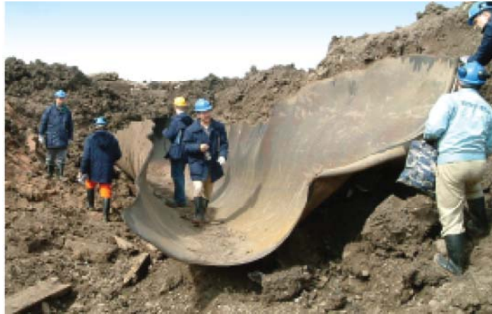
A running fracture – result of a test
