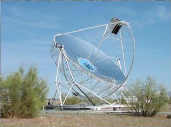
parabolic dish (SBP)
