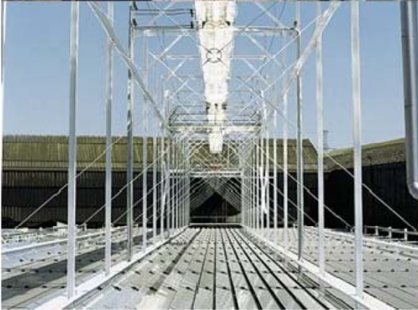
linear Fresnel (Solarmundo)
