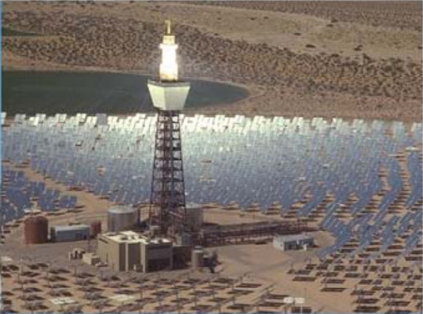
solar tower (SNL)
