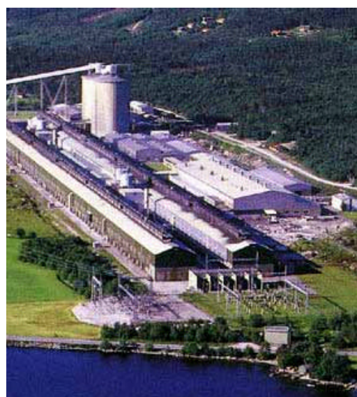
Exhibit 1. Primary Aluminium Reduction Plant
