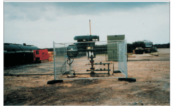
Coal bed methane test well at Sealand, Chester, UK. (Courtesy of Evergreen Resources)
