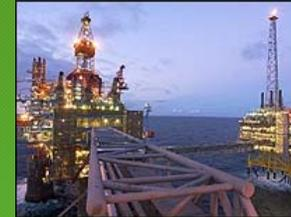
**Sleipner capturing and injecting 1Mt/y CO<sub>2</sub> since 1996**
