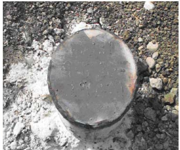
Capping surface casing
