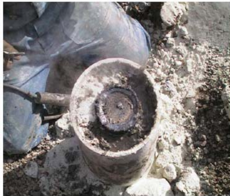
Capping production casing
