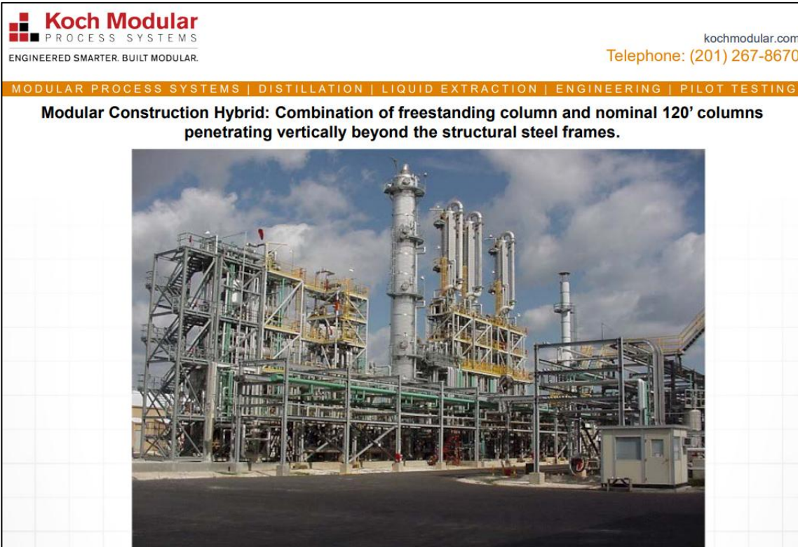
Fig. 2.14.4 Koch Modular – Hybrid Modular Construction [42]
