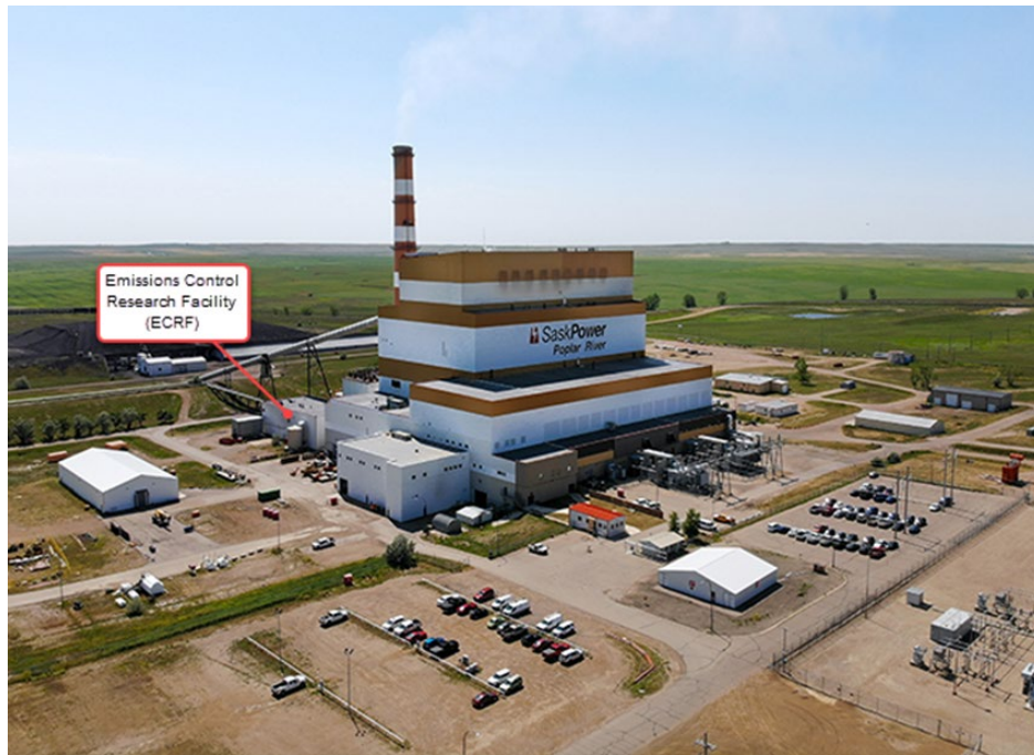
Figure-6: Emission Control Research Facility (ECRF) at the Poplar River Power Station
