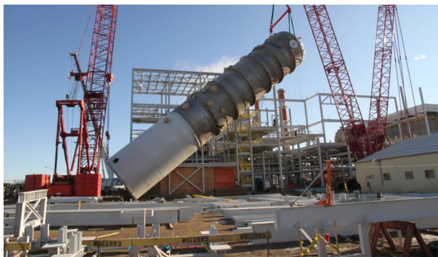
Figure-4: Prefabricated CO 2 Stripper
