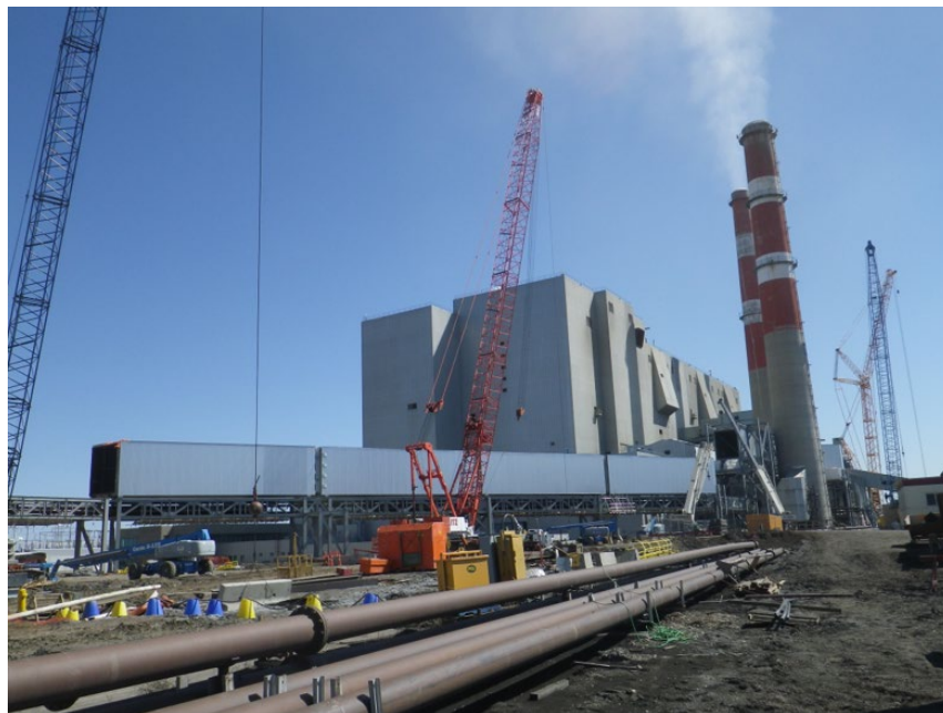
Figure-3: Prefabricated Flue Gas Ducting
